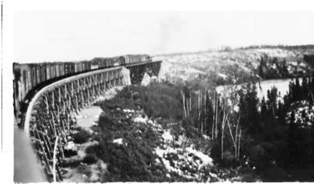
Photo 10: Nelson River Manitou Bridge c1929 (Photo Credit: FFCA 37 , Photo No. 1028720).
