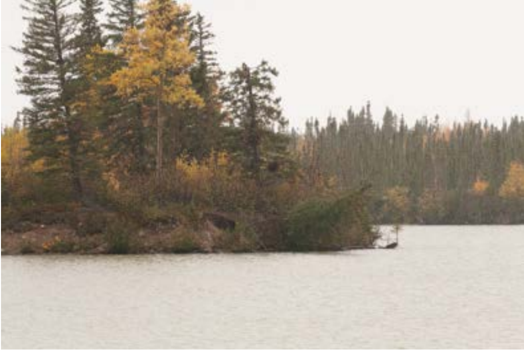
Photo 44: The shores just behind (upstream) Limestone GS, September 2016. (Photo Credit: Victoria Grima)
