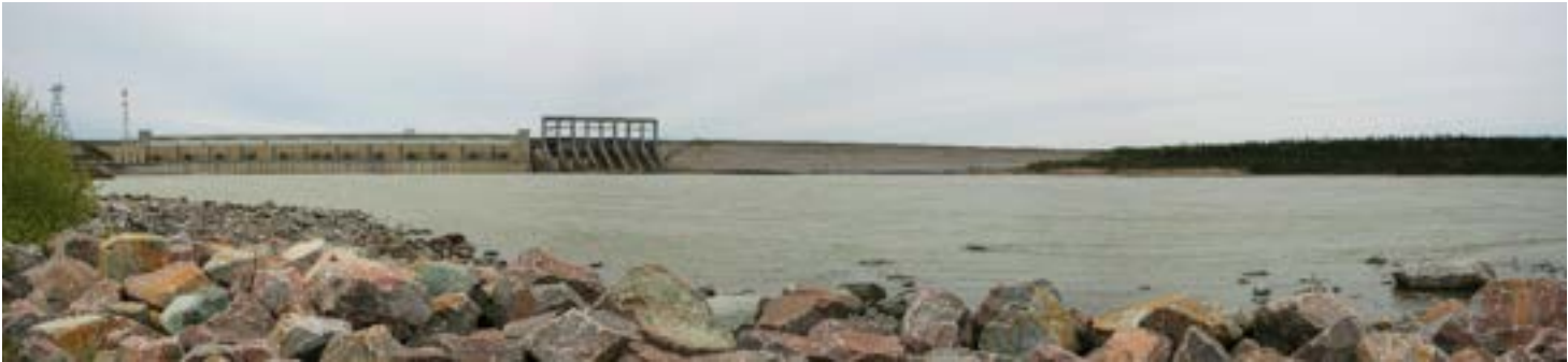
Photo 30: Kettle Hydro-electric Generating Station, June 2016. (Photo Credit: Victoria Grima)
