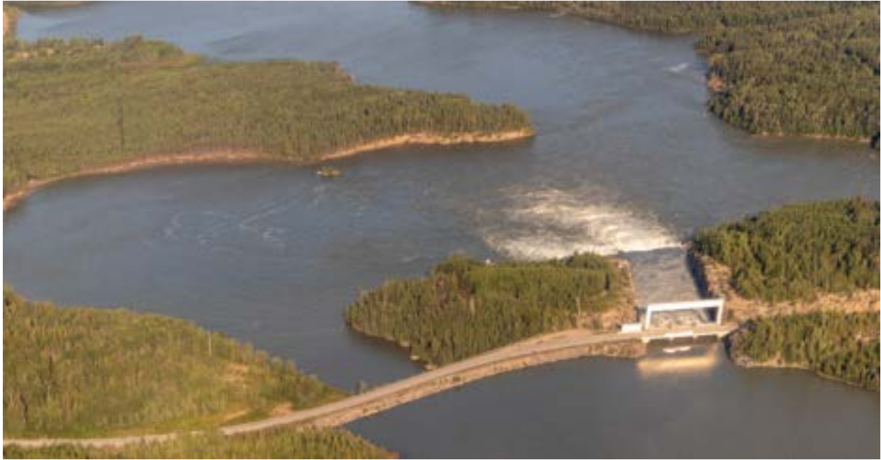
Photo 61: Notigi CS and the impounded original outlet, August 2019. (Photo Credit: Victoria Grima)
