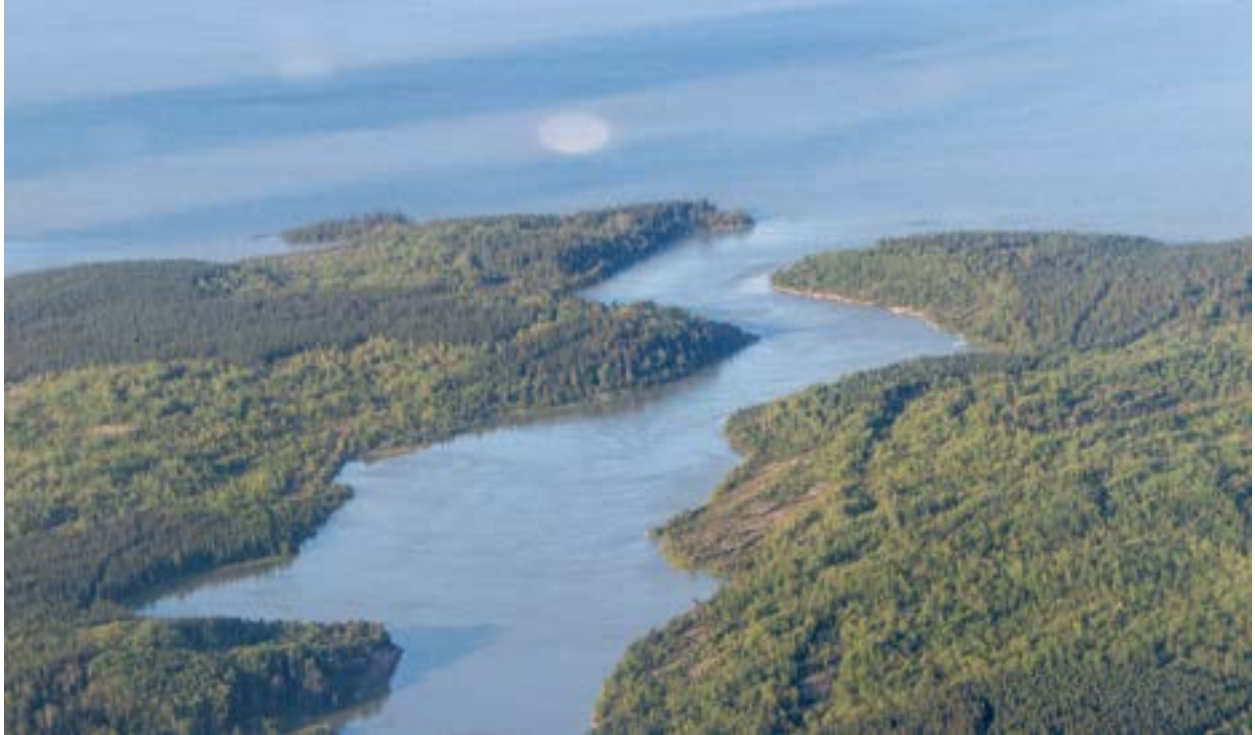
Photo 52: Aerial view of the Diversion Channel, August 2019. (Photo Credit: Victoria Grima)
