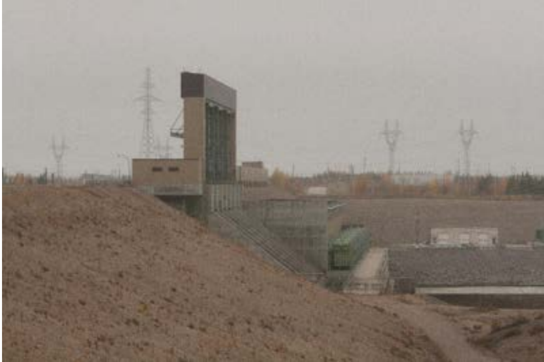
Photo 42: Limestone Hydro-electric Generating Station, September 2016. (Photo Credit: Victoria Grima)
