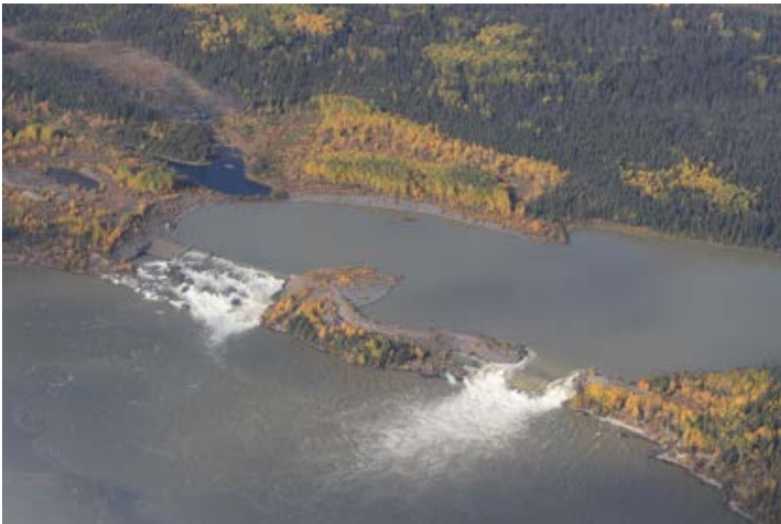
Photo 105: An aerial view of the reengineered Manasan Falls, location on the lower branch of the Burntwood River, August 2019. (Photo Credit: Victoria Grima)
