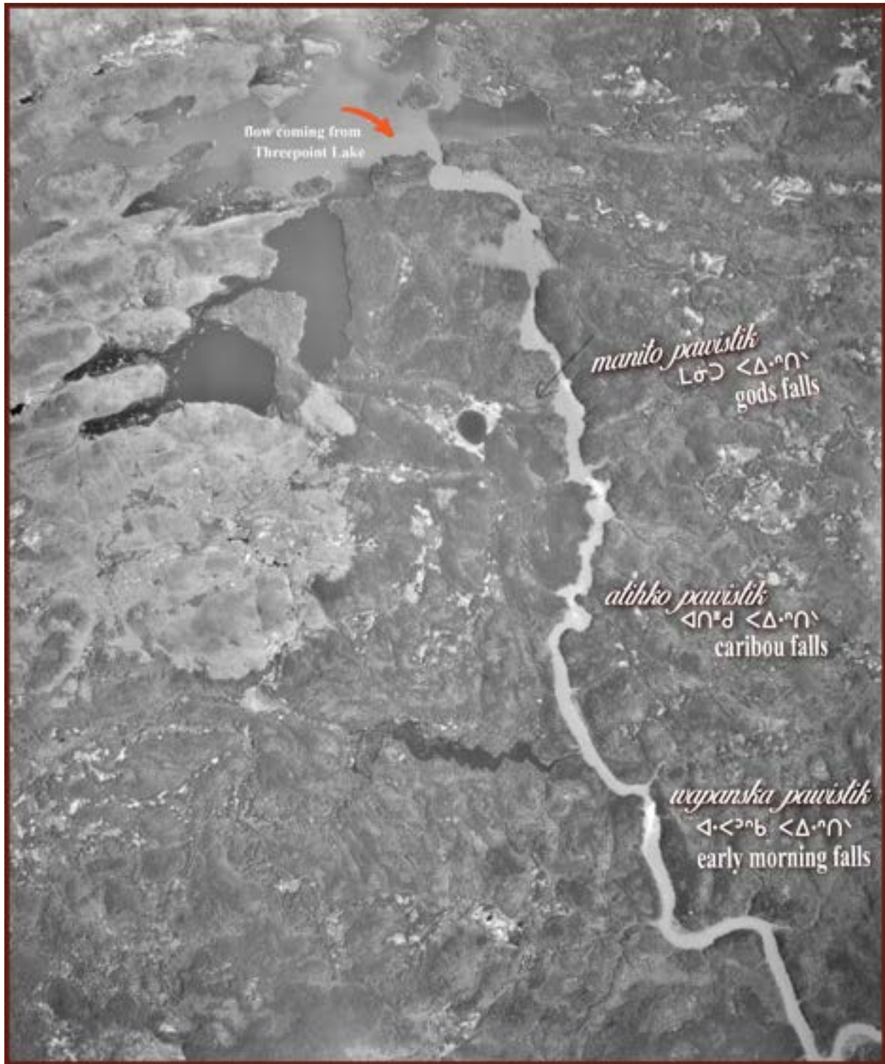
Photo 76: The branch that connects Threepoint Lake with Wuskwatim Lake in 1978. It was observed that the islands which once characterised the falls of caribou and early morning were completely submerged due to the operations of Notigi CS. (Acquired from NAPL, Roll No: A24936, Photo Nos: 0165)
