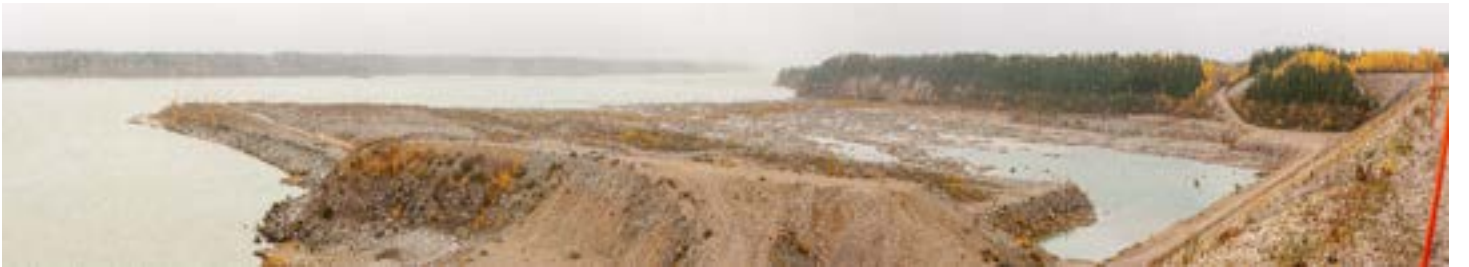
Photo 40: Limestone Hydro-electric Generating Station Cofferdam, September 2016. (Photo Credit: Victoria Grima)
