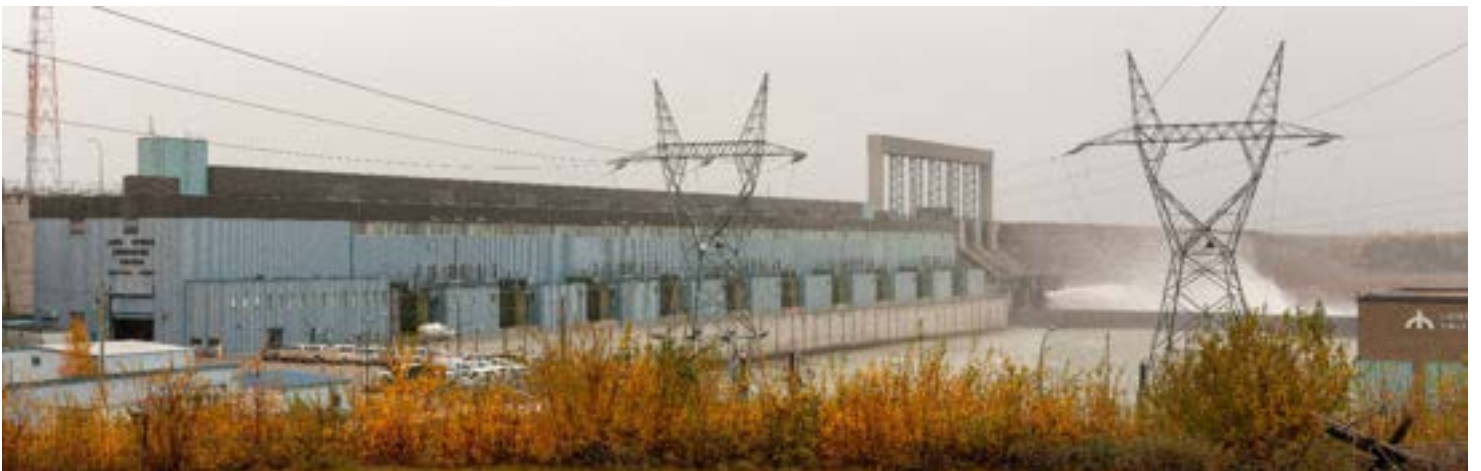
Photo 34: Long Spruce Hydro-electric Generating Station, September 2016. (Photo Credit: Victoria Grima)
