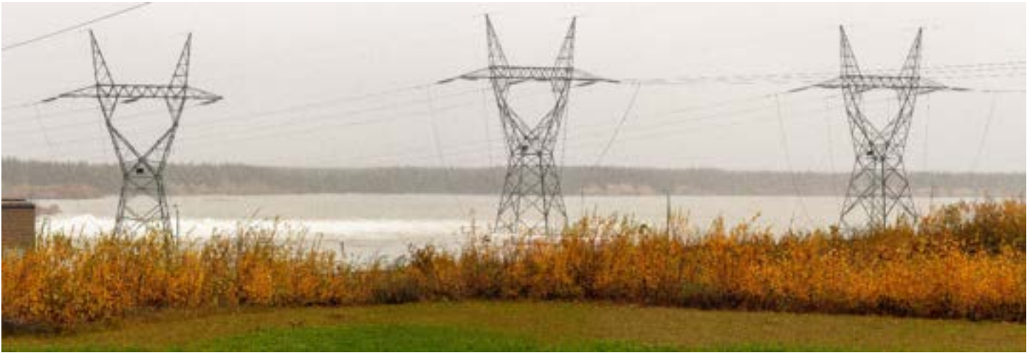
Photo 35: Downstream section from Long Spruce Hydro-electric Generating Station, September 2016. (Photo Credit: Victoria Grima)
