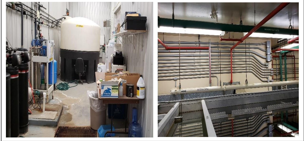
Figure 32: Water Bottling plant in Keeseekoowenin Ojibway FN (left).
